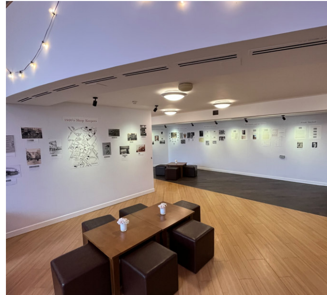
Ground Floor Entrance services includes radiator heating along with sidewall and linear diffusers for ventilation. Down lights and surface mounted light fittings.
